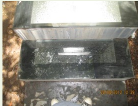
Glass window to monitor solids pit
