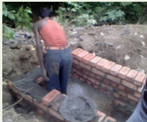
Pits under construction
